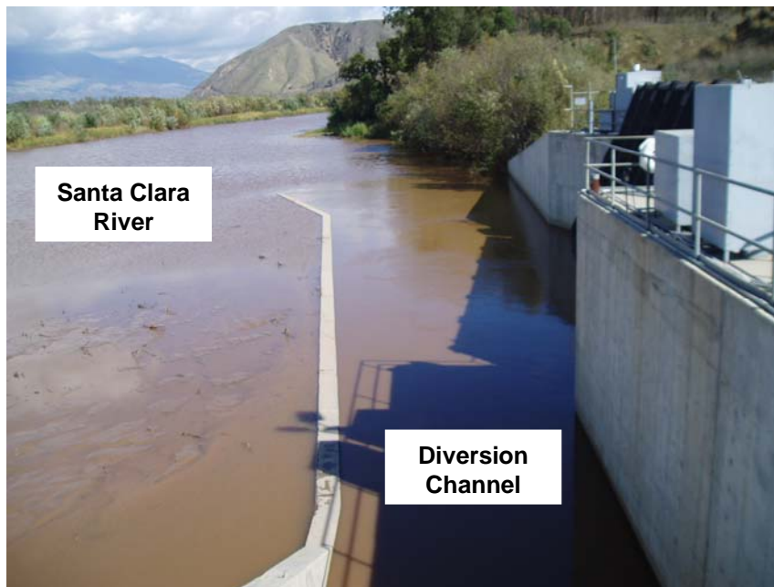
Figure 11: ME-SCR Freeman Diversion Dam (Facing Upstream)
