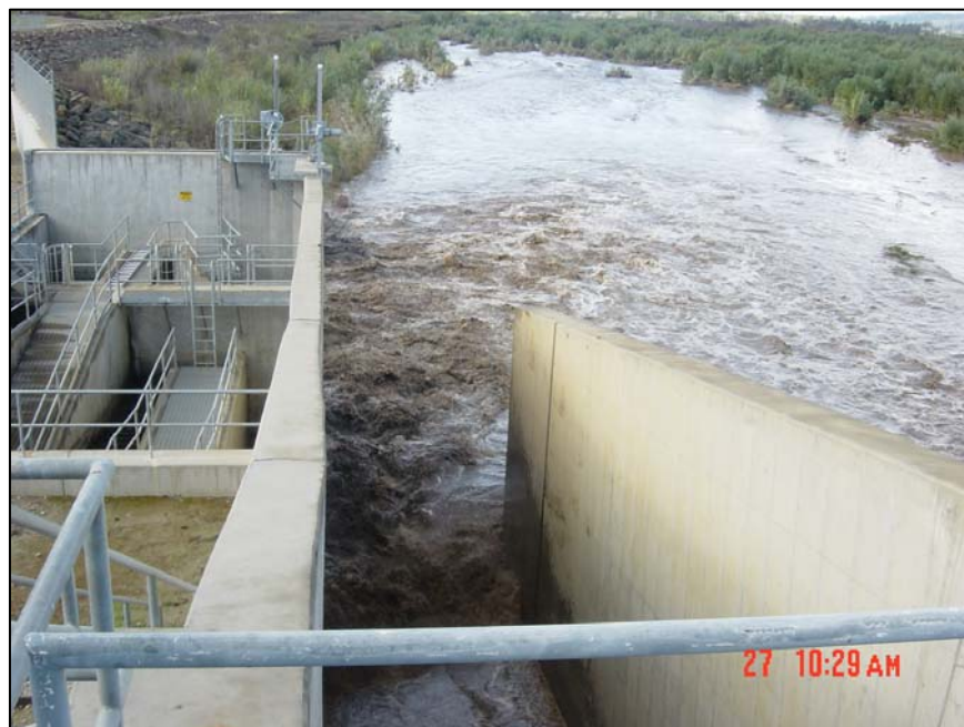
Figure 13: River Diversion Gate (Facing Downstream)
